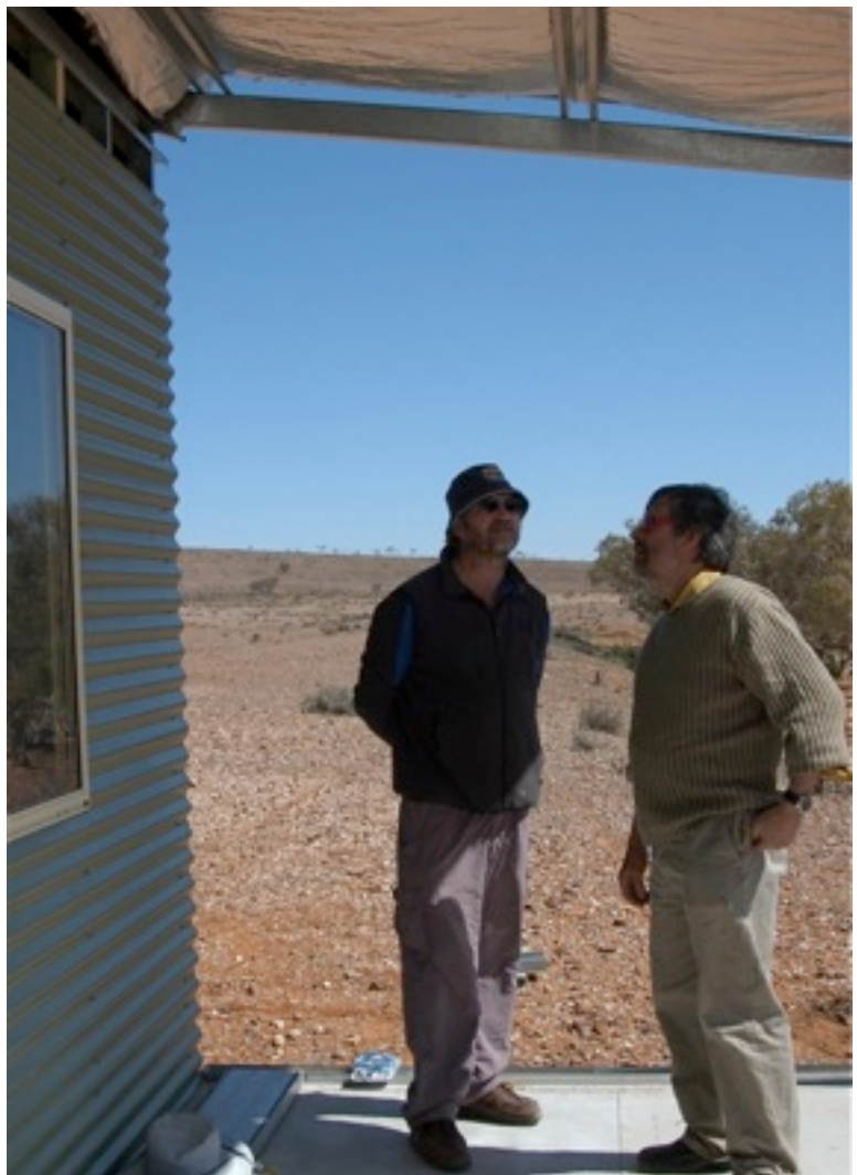
Idris and Dr David Croft inspecting construction work on the new Postgraduate Studio at Fowlers Gap.
