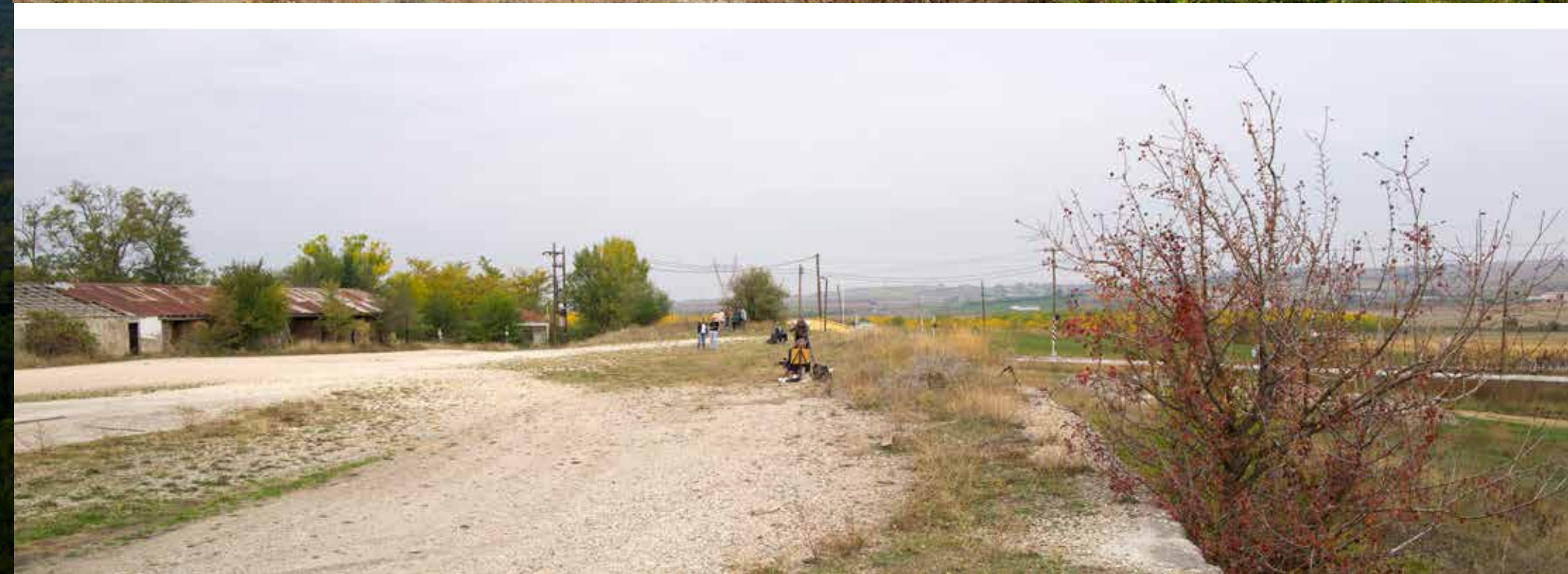
top: The bridge over the Pinios River near Tempe Gorge, Greece, was the site of a spirited defence by Major General A S 'Tubby' Allen's 16th (Australian) Brigade and elements of the NZ Division on 17-18 April 1941. Photo: Robert Linnegar.
